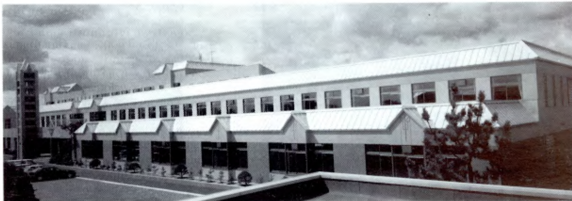
Hakodate: new classrooms and bell-tower.
