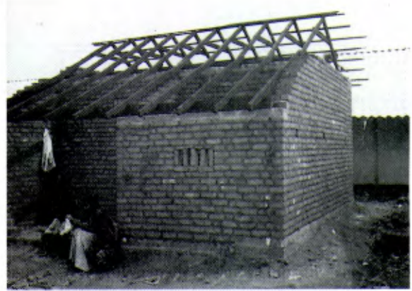
St Joseph's Boys' Village: a new house has just been built. All that's missing is the roof.
