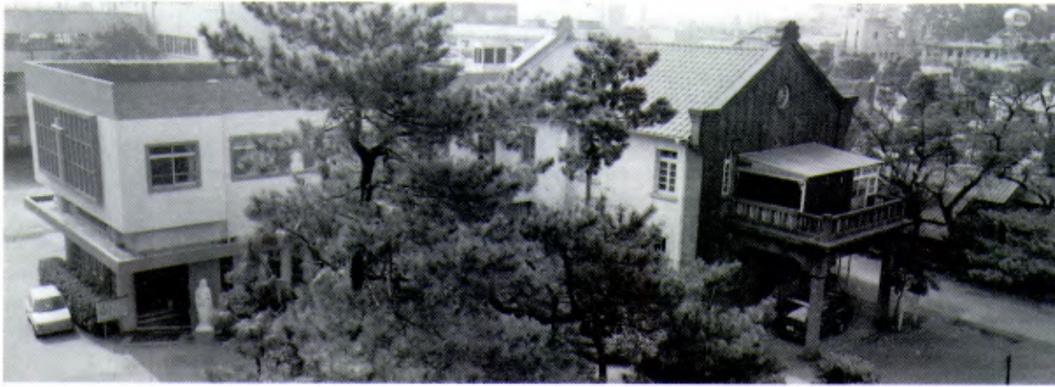
Kagoshima: the Brothers' house. The left part was built in 1963, the right, in 1930.
