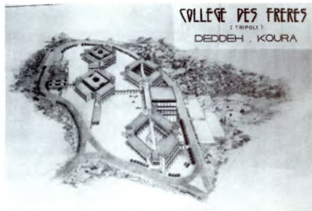
General view of the school at Deddeh Koura.
