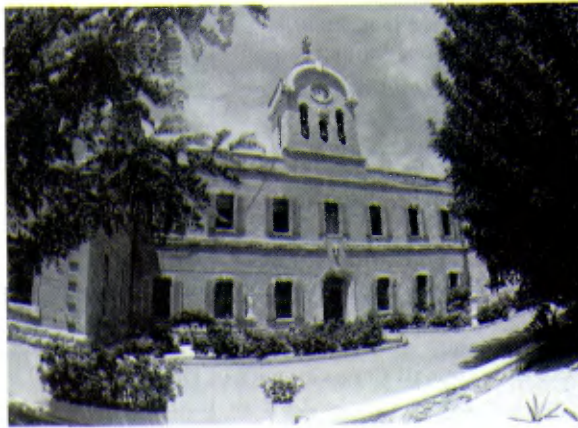
Bethlehem University: the original building.
